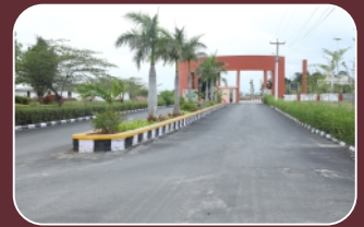
60ft, 40ft & 30ft BT Roads
